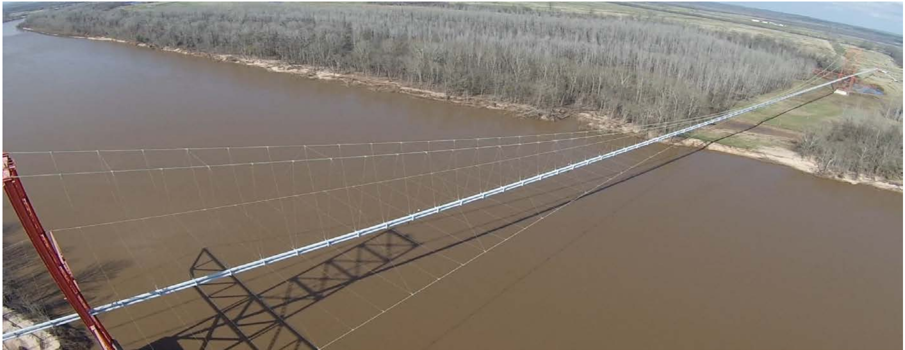
Aerial photo of a pipeline bridge crossing the Red River.
